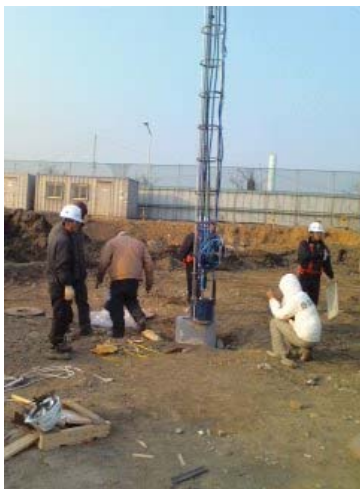
Installing the O-cell
