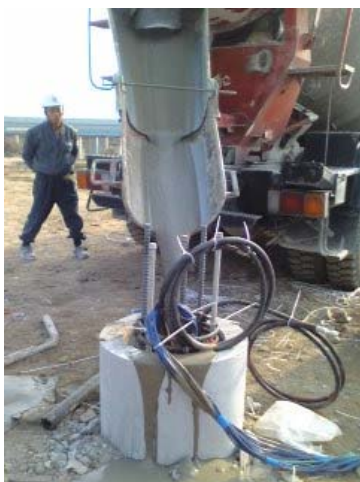
Concreting the PHC pile
