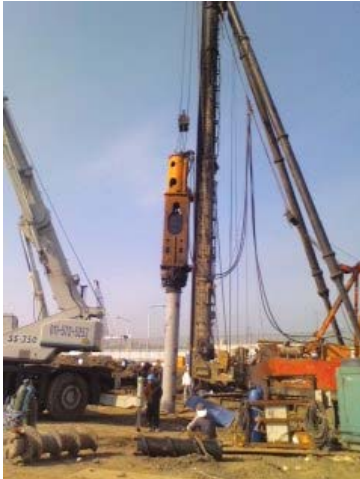
Driving the PHC Test Pile
