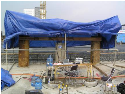
Pile Testing in Progress
